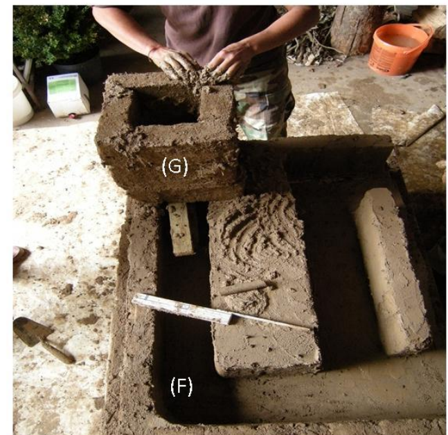
6: Base de la chimenea (Mod.1)
